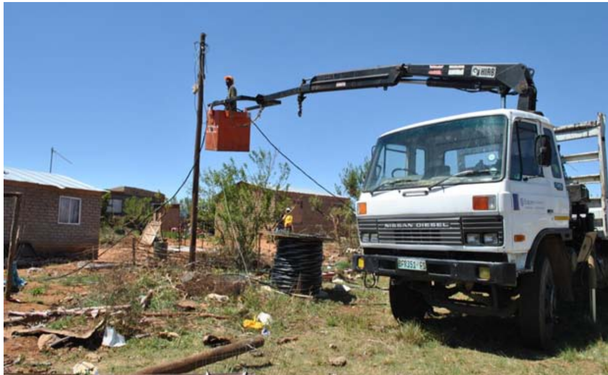
Eskom reinstalling electric cables destroyed during the tornado
